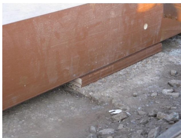
Figure 4. Recycled FFU production waste (K-FFU) between FFU sleeper and thrust bearing.
